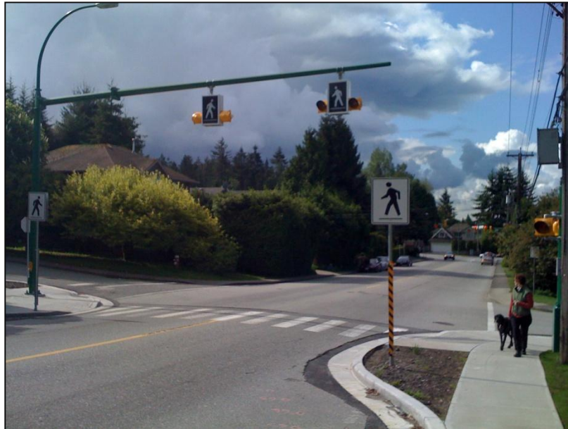
Figure 21 – Crosswalk with Flashing Lights
