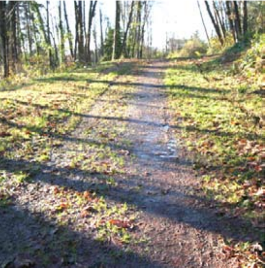
4 Standing water on the trail indicates potential drainage issues.
