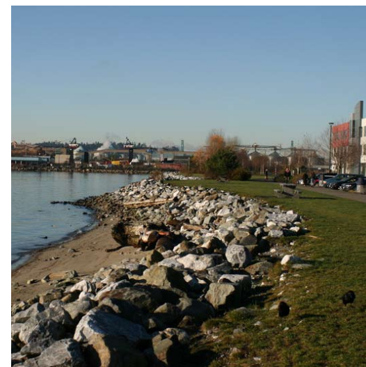
1 Typical waterfront treatment; riprap and turf.
