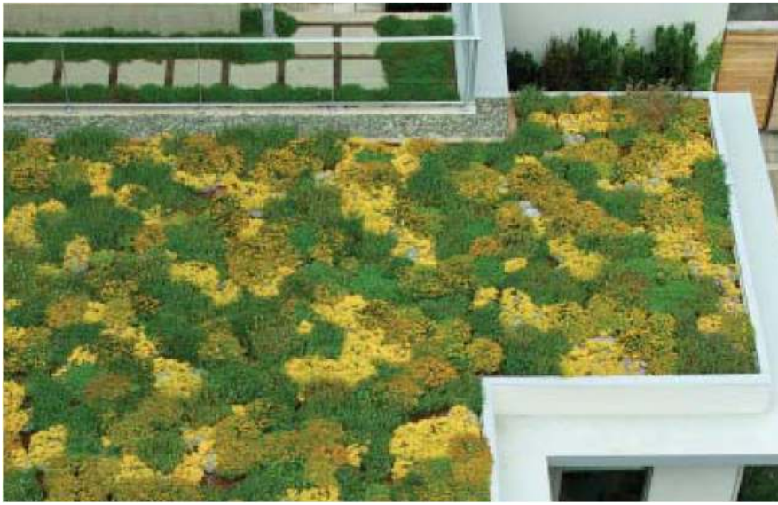
Figure 7. Green roofs can help reduce the rate and volume of stormwater run-off and improve water quality
