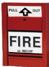
Pull stations are typically located at the exit doors from each floor level and when activated will sound the bells and send a signal to the Fire Department through the monitoring station.
