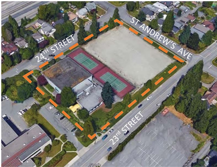
AERIAL VIEW OF MICKEY MCDUGALL SITE, SW CORNER (FIG 4)
