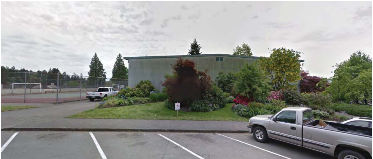
LANDSCAPING AT THE NORTH END OF THE MICKEY MCDUGALL FACILITY (FIG 5)
