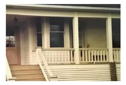
Cancel one of the two front doors on the facade (the central opening survives from before the side porch was enclosed and an additional front door was introduced in the 1930s) to allow for better layout on the interior. Replace the door opening with a window opening.
