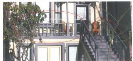
Code compliant balustrade, circled in red; the glass inserts are barely visible. A metal handrail installed on the staircase would also be a reversible and acceptable solution.
