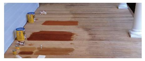
Photo shows a historic tongue and groove porch surface in the process of being refinished and restained. Note the boards are perpendicular to the house while the nosing piece is parallel to it.
