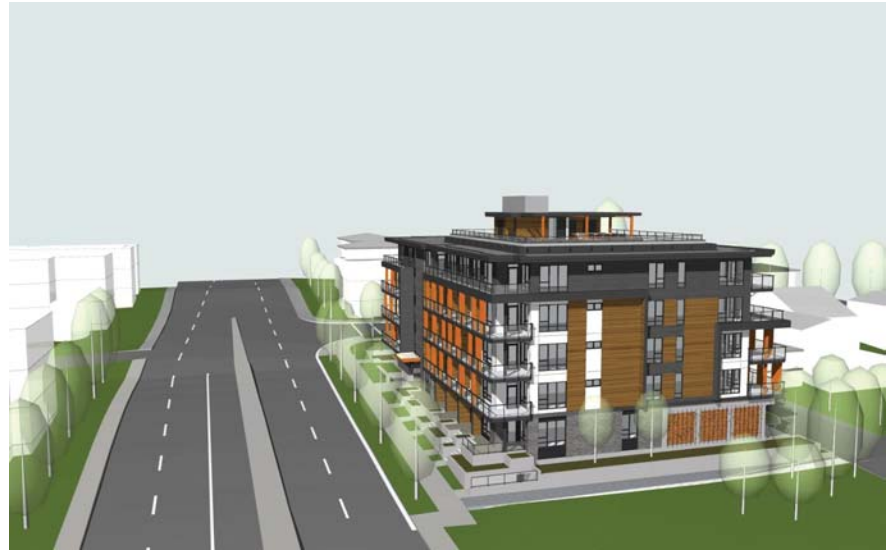
VIEW NORTH - ALONG LONSDALE AVE
