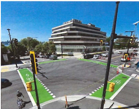
Green mobility lane markings are added to the Chesterfield protected intersection.
