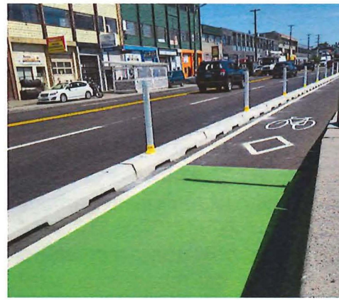
Curbs are placed to separate parking spaces and the mobility lane on the 200 Block East.
