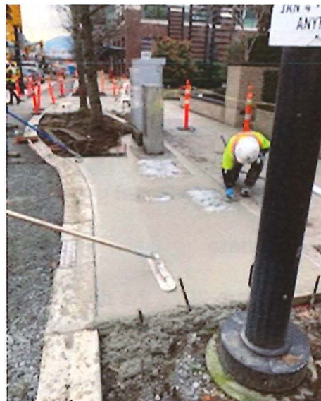
Temporary surfaces are replaced with final concrete sections.
