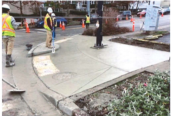
Temporary surfaces are replaced with final concrete sections.
