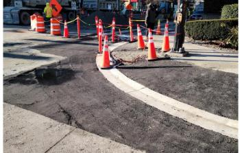
Interim asphalt surfaces are placed at St Georges to ensure a safe sidewalk and mobility lane condition for all. This photos shows work in progress and the completed surface will be flush to eliminate hazards.
