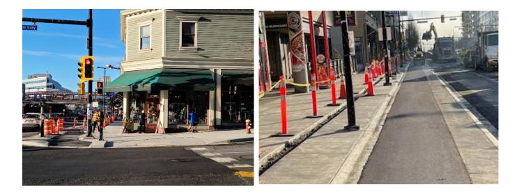
Fresh sidewalk is installed on the northwest corner of Lonsdale and Esplanade, the City's busiest pedestrian corner. Pedestrian access is maintained around the active work area.
