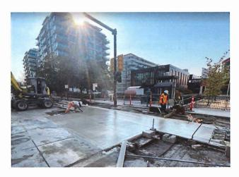
The midblock crossing is poured over the underground structure repair between Lonsdale and St Georges. This crossing is now open to pedestrians again.
