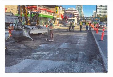
Base repair works completed throughout the Chesterfield intersection. This proactive repair work will improve the life span of the new asphalt.
