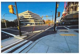
New completed protected intersection corner at Chesterfield and Esplanade. The addition of pavement markings helps delineate walk spaces from mobility lane spaces. The team is already seeing positive behaviour shifts as the legibility of the design emerges more completely.
