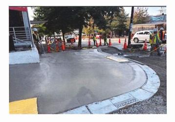
The new sidewalk is poured at the southeast corner of Lonsdale and Esplanade. Paving for the mobility lane will be completed this week. When complete, eastbound cyclists and mobility devices users will have a protected travel space from 3<sup>rd</sup> Street to St. Georges.
