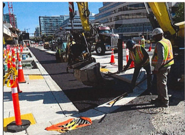
Fresh mobility lane paving finishing up on the section between Rogers and Semisch on the north side of Esplanade.
