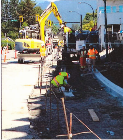
New mobility lane and vehicle lane curbs are installed on Forbes.
