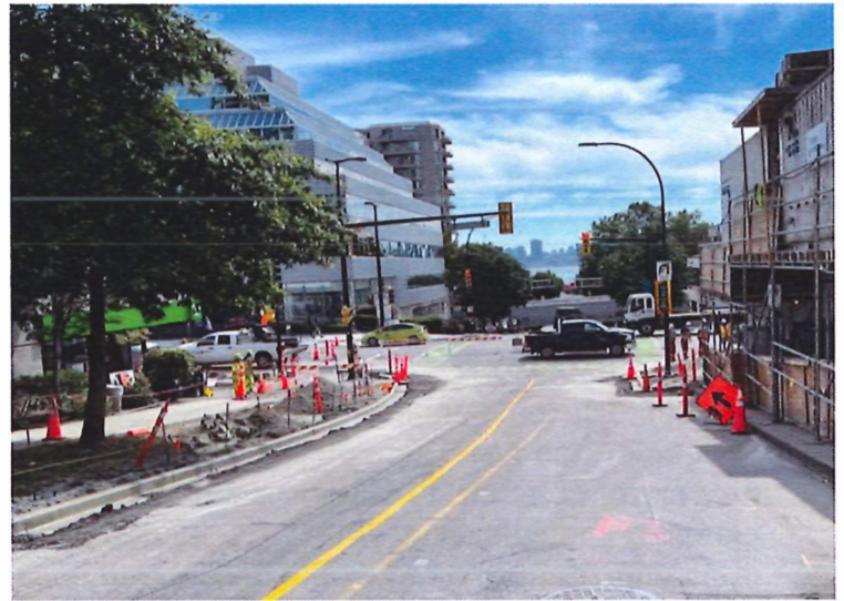
Temporary line markings and new curbs are placed on Chesterfield. The existing painted lanes on Chesterfield will transition into protected space on the approach to Esplanade.
