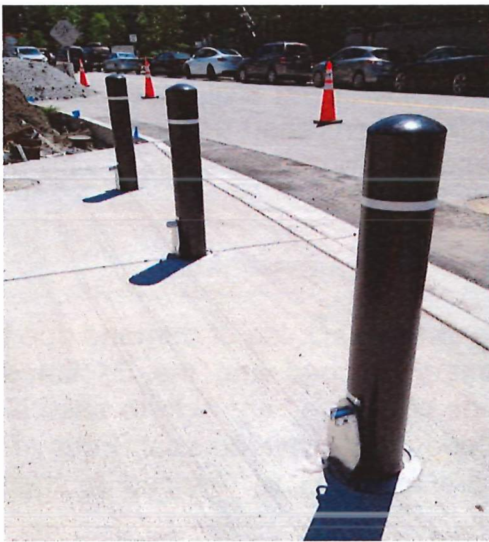
Removable bollards are installed at the new Mahon closure to maintain emergency services access while limiting vehicle traffic outside Alcuin College.
