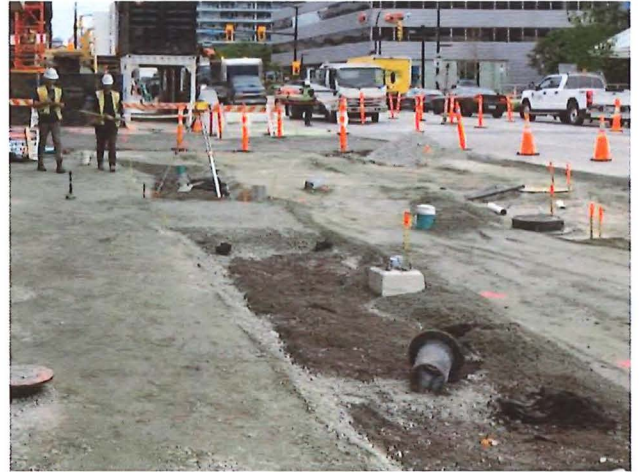
Preparation of soil and drainage for new trees and planted areas between Chesterfield and Rogers
