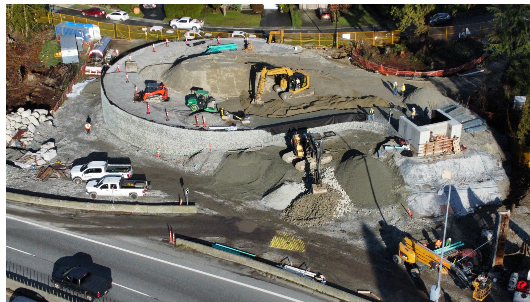
North approach path and abutment
