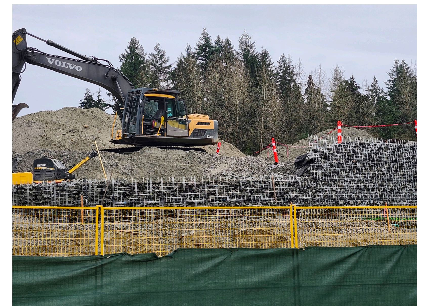
North side MSE retaining wall
