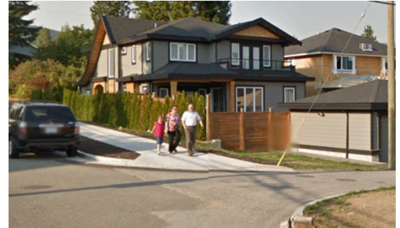
▲ Ridgeway Ave. north of E 10 th St. with newly installed sidewalks
