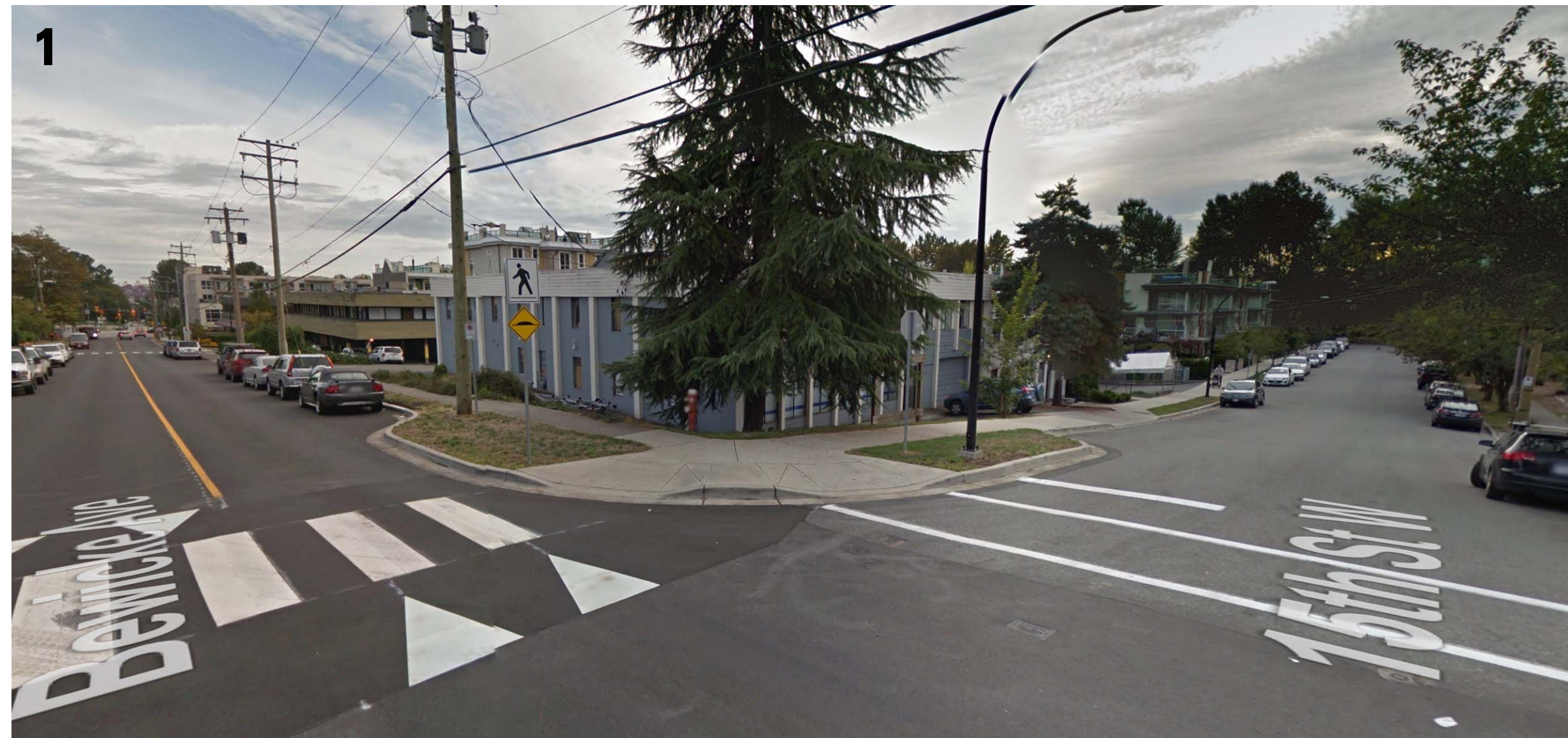
VIEW TOWARDS SITE FROM NORTHEAST CORNER
