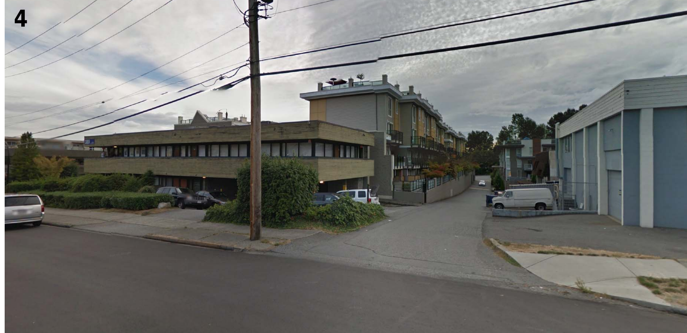
VIEW TOWARDS LANE FROM SOUTHEAST CORNER
