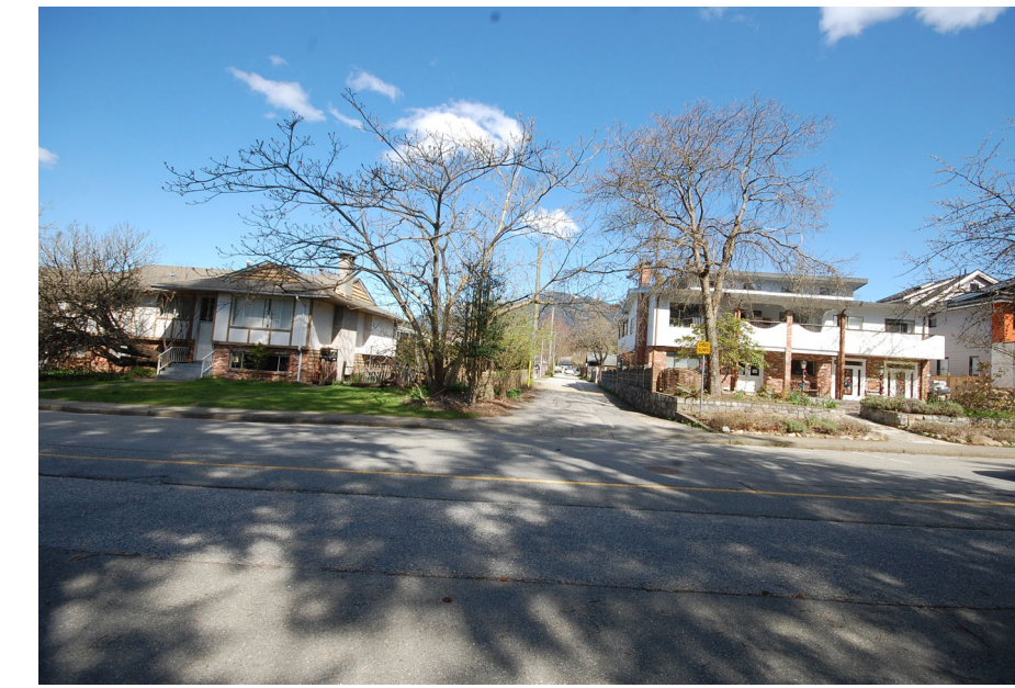
North Side of West 19th St.
