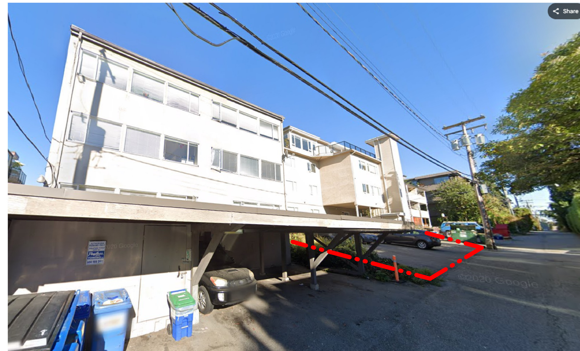
4. EXISTING SITE - 321 AND 329 FROM LANE AT WEST P.L.
