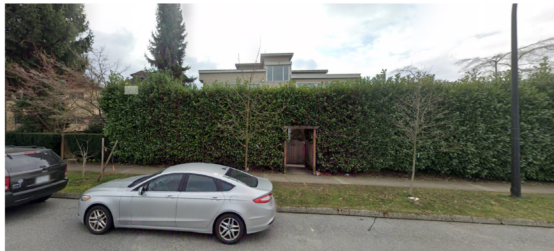
2. EXISTING SITE - 321 W 4TH STREET
