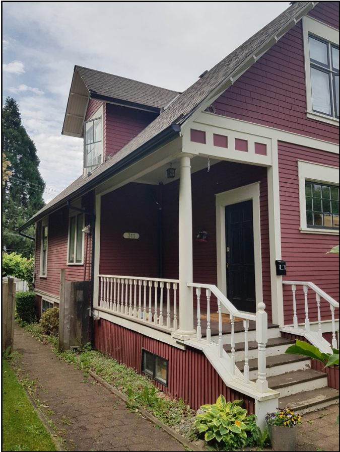
side view (east elevation)
