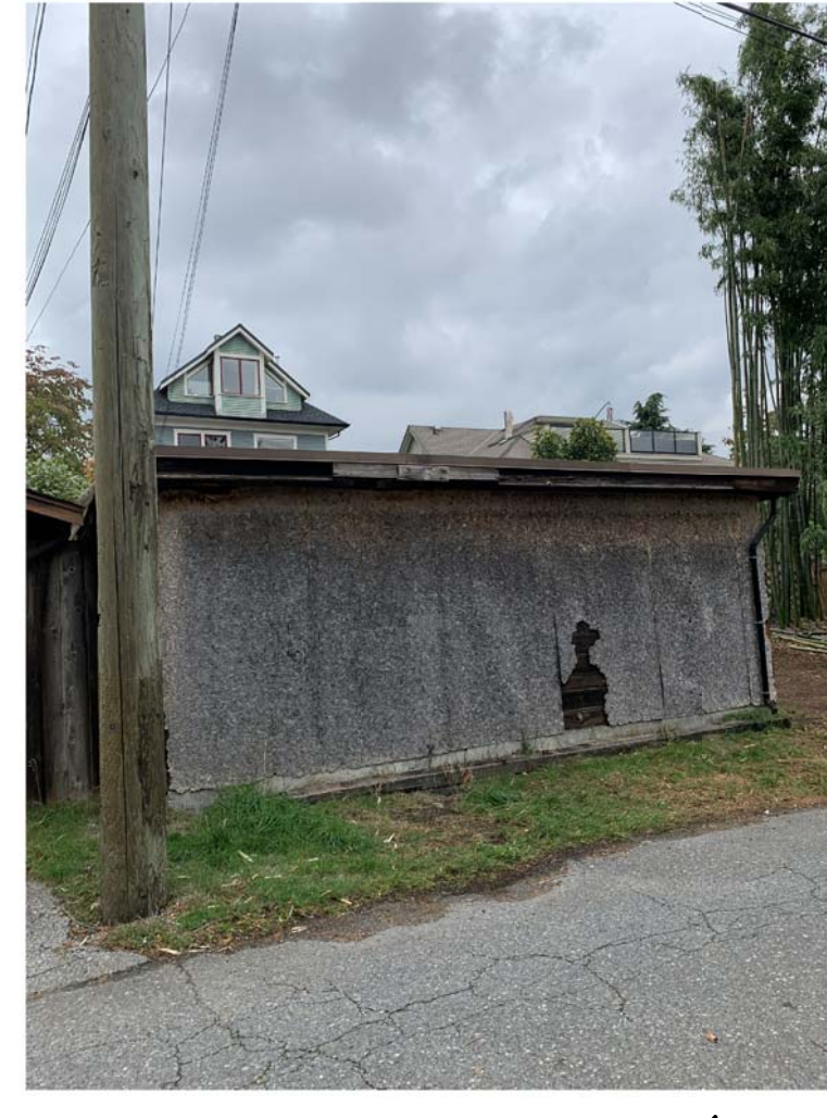
245 EAST 10TH EXISTING GARAGE (FROM LANE)
