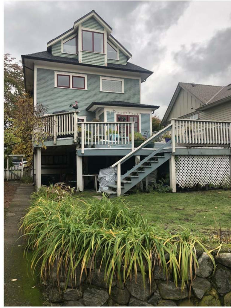
245 EAST 10TH REAR FACADE
