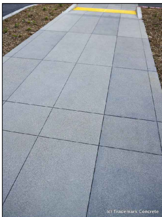
SAW CUT CONCRETE
