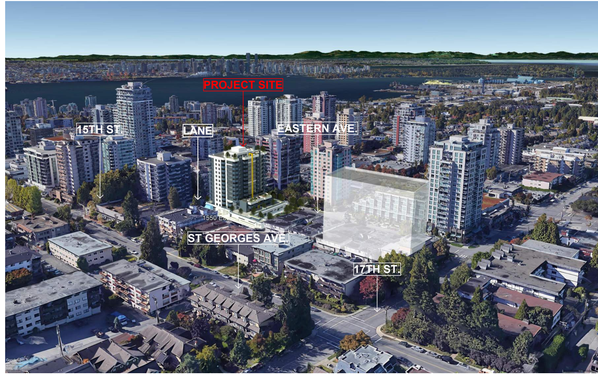
VIEW FROM NORTH EAST
