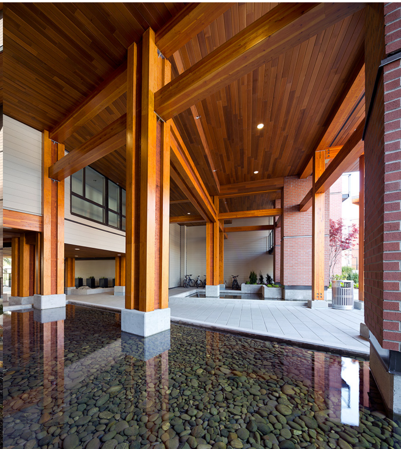
EXPOSED WOOD STRUCTURE AND SOFFITS
