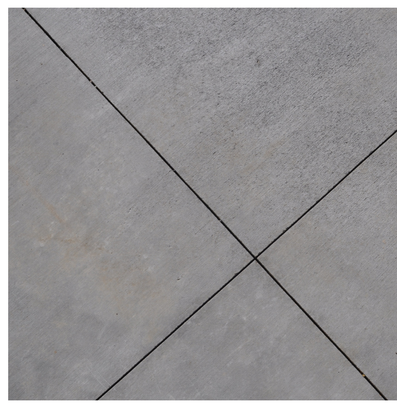
CIP CONCRETE PAVING
