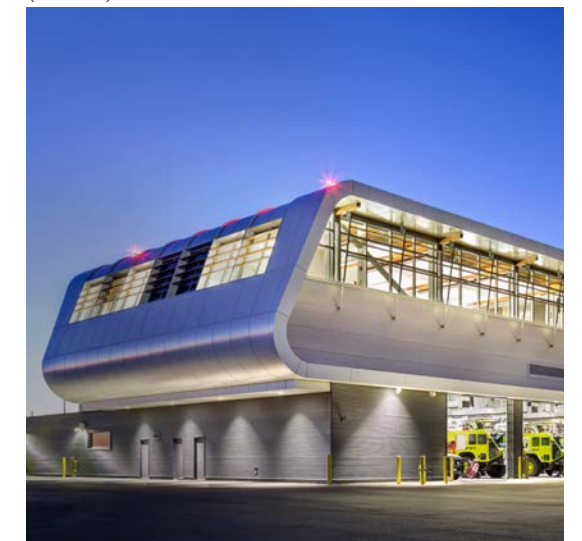
YVR AIRSIDE OPERATIONS BUILDING (Francl)
