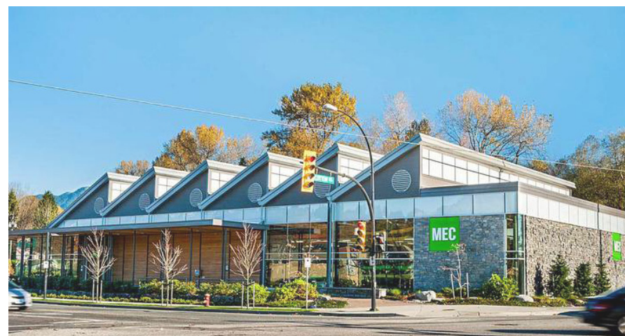
MEC NORTH VANCOUVER Retrieved Mar, 29, 2021 from: https://russ-tresoor-mg5s.squarespace.com/mec-store/
