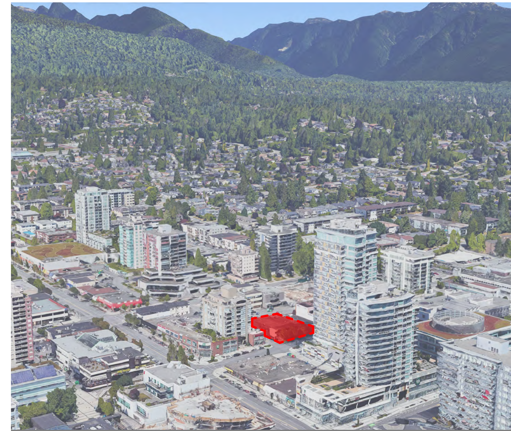
SITE - VIEW NORTH OF SITE TOWARDS MOUNTAINS
