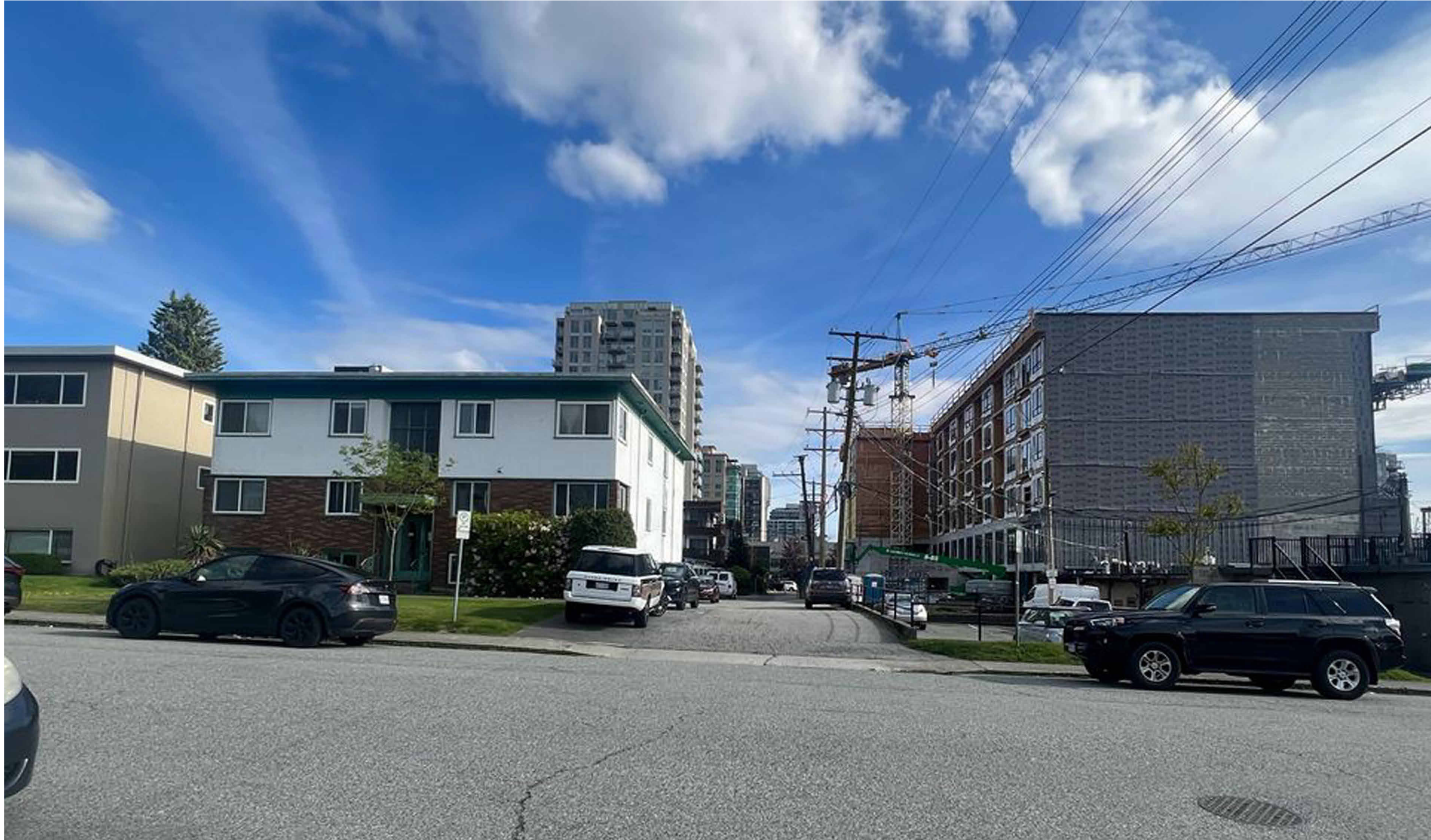
18TH STREET EXISTING STREETSCAP
