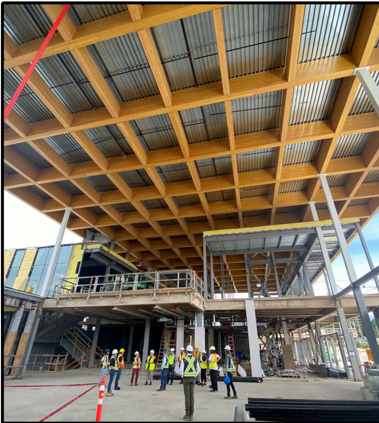
Final stages of mass timber installations
