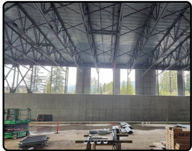
Arena under construction
