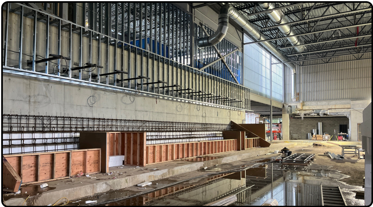
Construction of the arena bleachers
