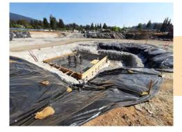
Shown is the foundation for the west tower crane, which will support construction until completion.
