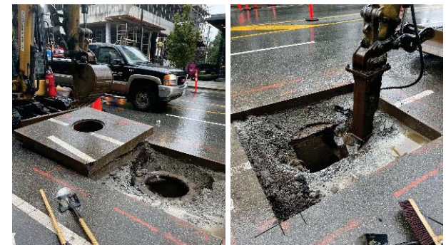
▲ East 13 th Street sanitary decommissioning
