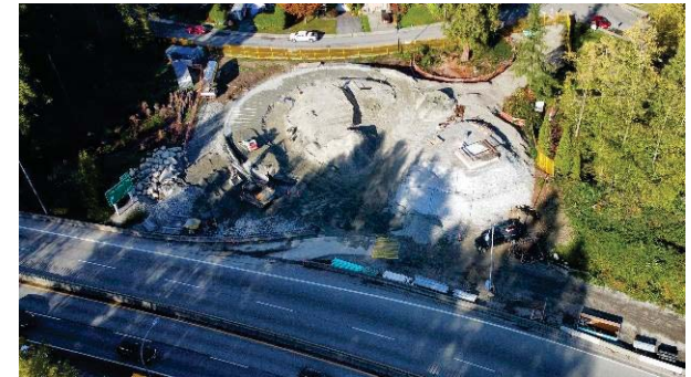
▲ North abutment of Casano-Loutet overpass under construction [2025]
