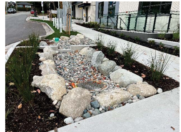
▲ Raingarden installation at St Patricks & East 3 rd [2025]
