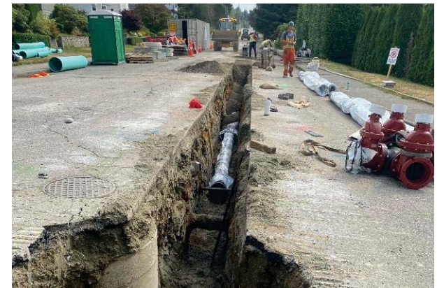
▲ West 27 th St. water main replacement [2024]
