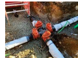
▲ 23 rd St. & St. Andrews water main replacement [2021]
