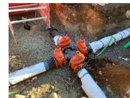
▲ 23 rd St. & St. Andrews water main replacement [2021]
