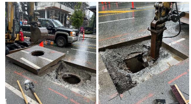
▲ East 13 th Street sanitary decommissioning
