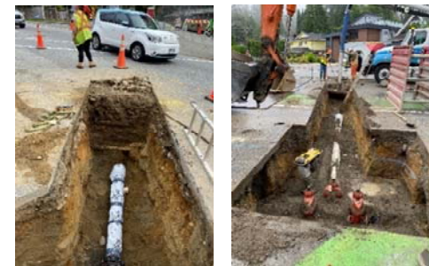
▲ Larson Rd. water main replacement (Bewicke & Larson and Westview & Larson segments shown) [2024]
