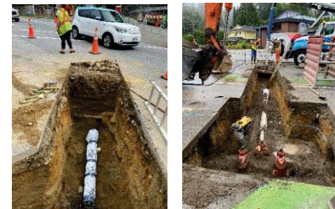
▲ Larson Rd. water main replacement (Bewicke & Larson and Westview & Larson segments shown) [2024]
