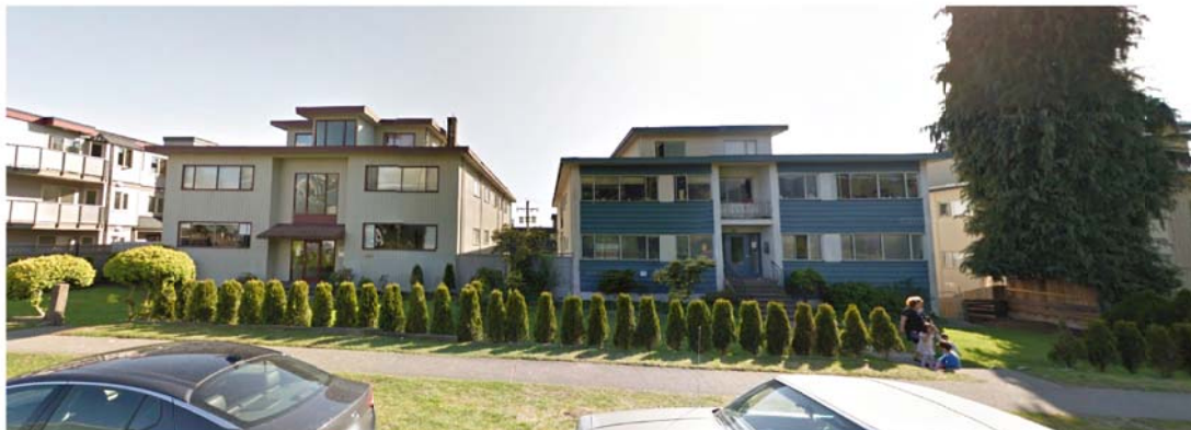
EXISTING BUILDINGS - 347 341 W 4TH ST
