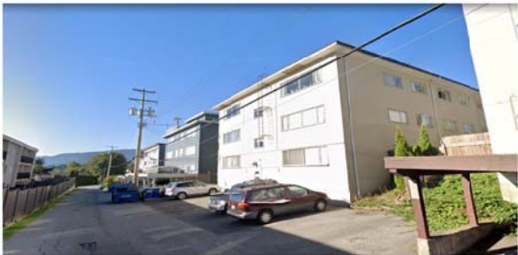
VIEW ALONG THE LANE AT 357 W 4TH ST
