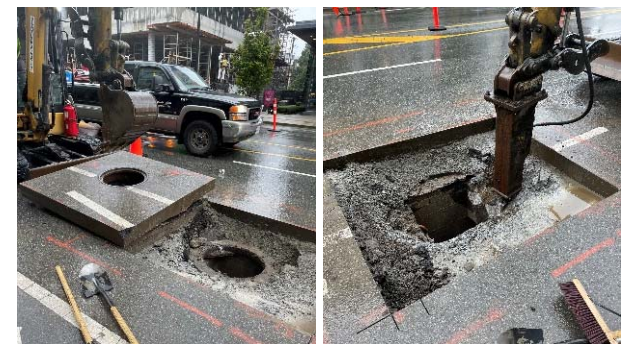
▲ East 13 th Street sanitary decommissioning
