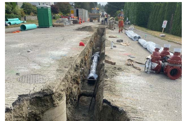
▲ West 27 th St. water main replacement [2024]
