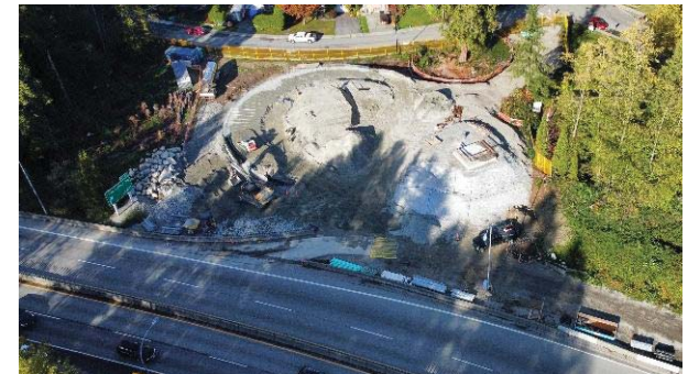
▲ North abutment of Casano-Loutet overpass under construction [2025]
