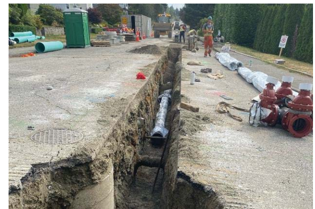
▲ West 27 th St. water main replacement [2024]
