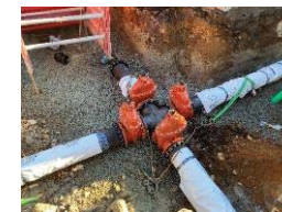
▲ 23 rd St. & St. Andrews water main replacement [2021]
