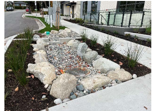
▲ Raingarden installation at St Patricks & East 3 rd [2025]
