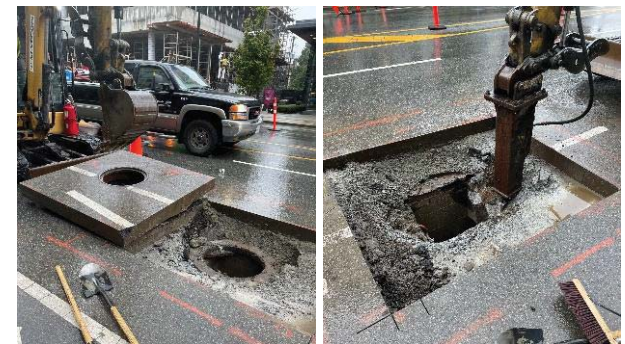
▲ East 13 th Street sanitary decommissioning
