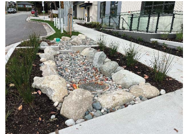
▲ Raingarden installation at St Patricks & East 3 rd [2025]
