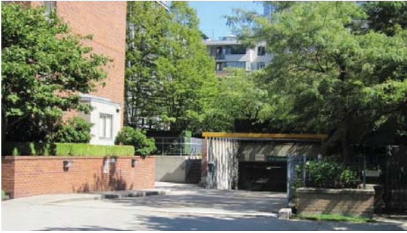
Recessed parking garage ramp
