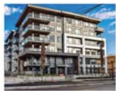
Lower Lynn (2023) • District of North Vancouver • 88 rental homes
