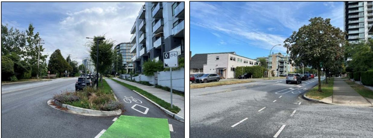
*Figure 11: (Left) Protected northbound mobility lane delivered by the adjacent development at Chesterfield and West 5th Street – looking north. (Right) Parking protected mobility lane at Chesterfield and West 8th Street - Looking north*
