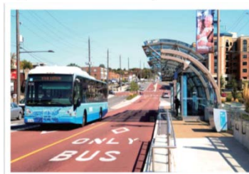
North Shore bus rapid transit at the front of the line, TransLink says
