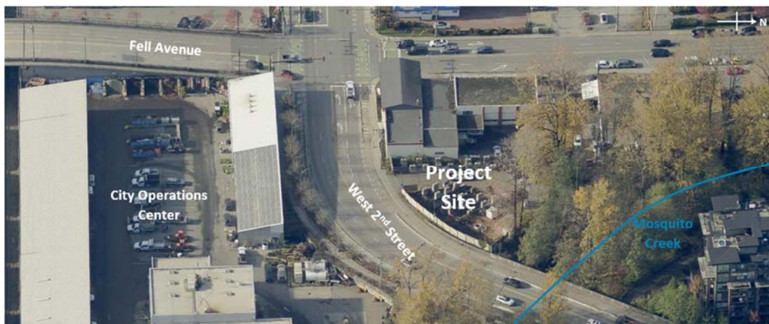
Figure 3 - Project Site for Sewer Heat Recovery Plant
