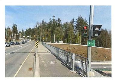
Cantilevered Pathway: Creation of a separate active mode facility connected to the existing interchange bridge.
