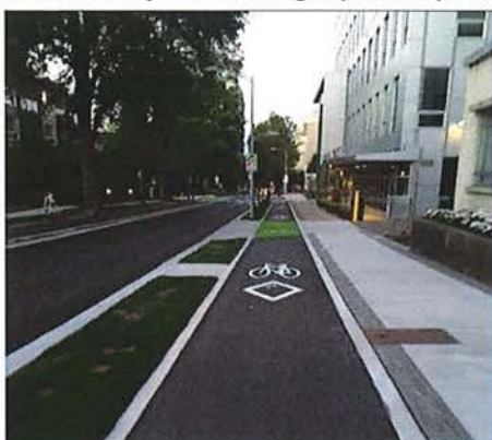
10 th Street, Vancouver: Directional off-road bike lanes next to sidewalk
