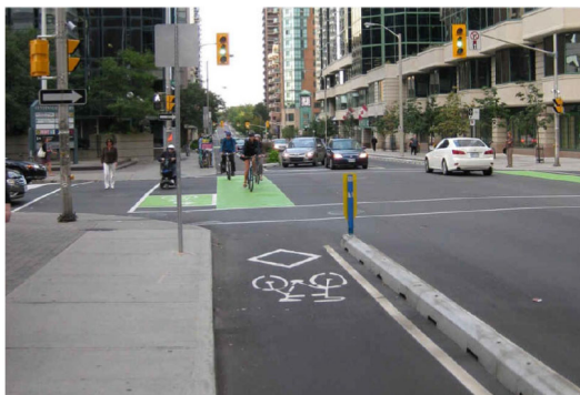
Laurier Avenue, Ottawa: Concrete barriers used to protect bike lane
