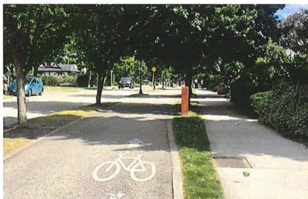
Abbott Street Greenway, Kelowna: Bi-directional off-road route with separation from the sidewalk
