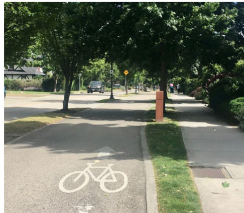
Abbott Street Greenway, Kelowna: Bi-directional off-road route with separation from the sidewalk
