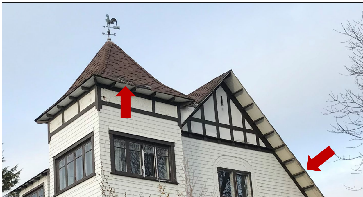
Fig. 13: Front view of the Knowles Residence at 328 W 14th Street, 2021. Note the missing shingles and signs of deterioration, pinpointed with red arrows. (Source: Leskiw)
