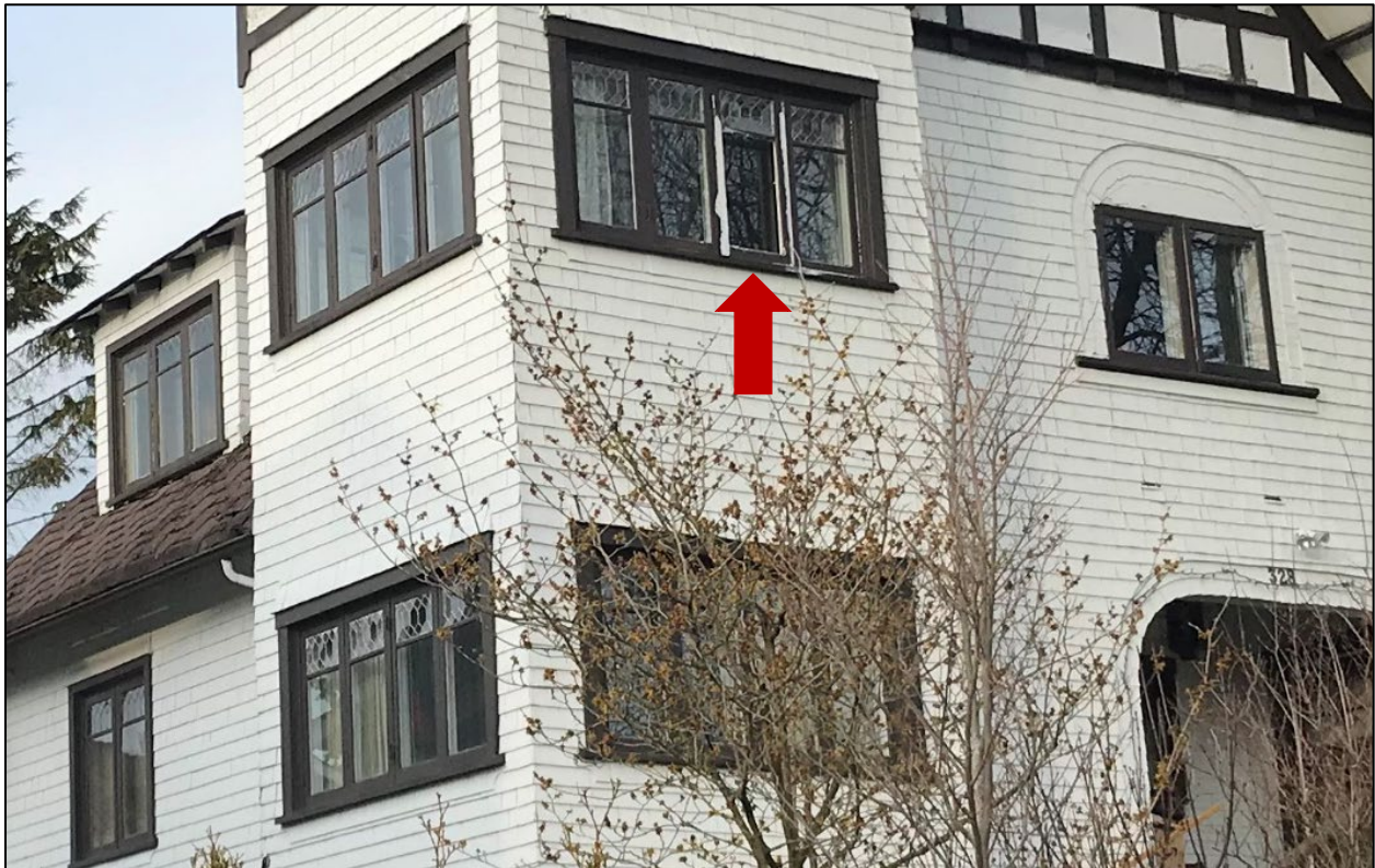
Fig. 15: Southwest corner view of the Knowles Residence at 328 W 14th Street, 2021, illustrating the largely good condition of its original windows, with leaded diamond patterned panes in the upper lites of the windows. (Source: Leskiw)
