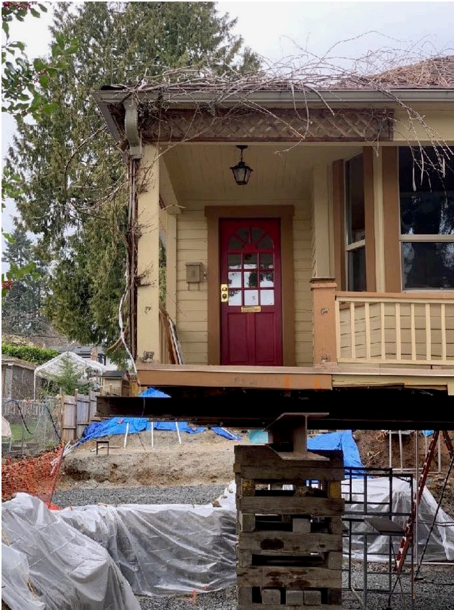
Current view of the subject house at its new location at 532 E 10th Street, temporarily sitting on cribs while a new foundation is excavated and poured.
