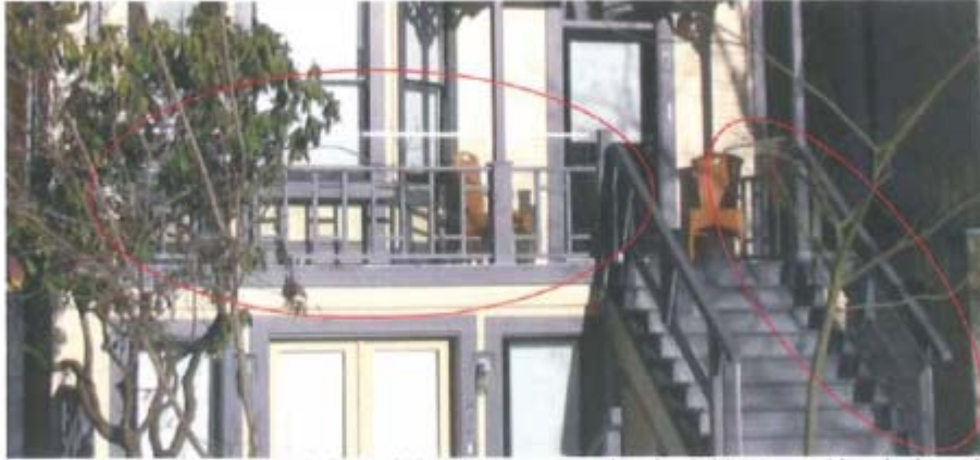
Code compliant balustrade, circled in red; the glass inserts are barely visible. A metal handrail installed on the staircase would also be a reversible and acceptable solution.
