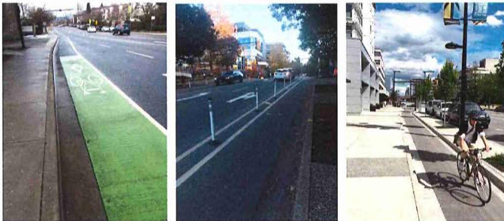
Figure 1: Examples of mobility lane infrastructure, from left-to-right: painted bicycle lane, paint buffered bicycle lane, and protected bicycle lane.
