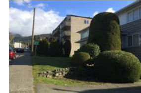
⑧ view from the sidewalk towards the site and the neighbor building
