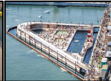
Arhus Harbor Bath Aarhus, Denmark - 2018
