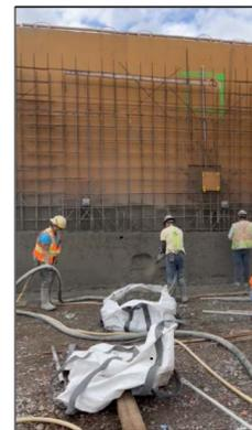
Concrete formwork, rebar and shotcrete work in April and May, 2023
