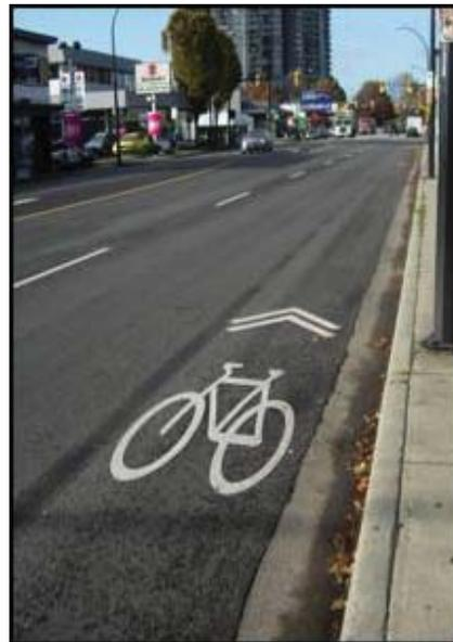
**FIGURES 3a & 3b: Single file travel on major or minor streets with "sharrow" markings to indicate to road users the safest position for cyclists:**
