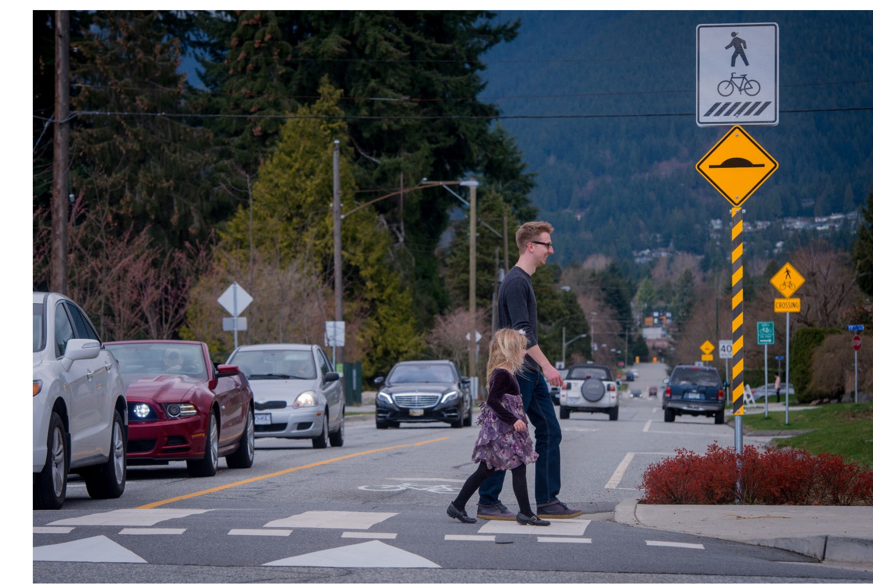
Raised Crosswalk: North Vancouver
