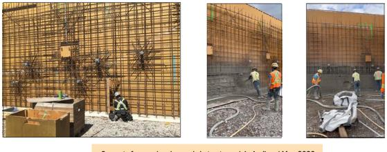
Concrete formwork, rebar and shotcrete work in April and May, 2023
